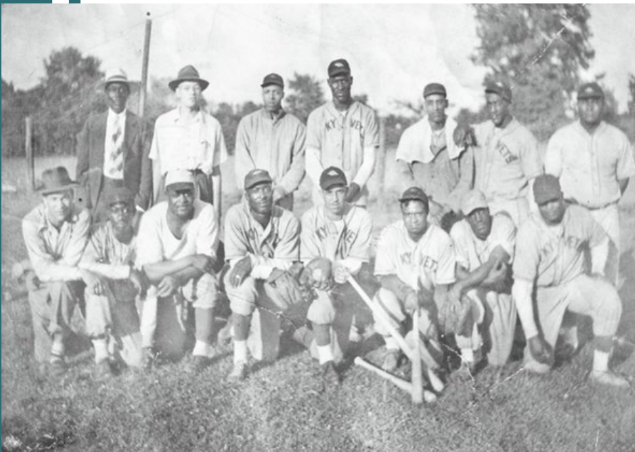
The City of Paris Waste Transfer Station is located on the tip of the West Side Neighborhood “peninsula” bound on three sides by Houston Creek. Prior to 1965 the “dump” site was formerly known as Riverside Park, a place where folks gathered from far and wide to play baseball and other organized sports. Photo Source: Bourbon County Citizen, May 6, 2021 edition
